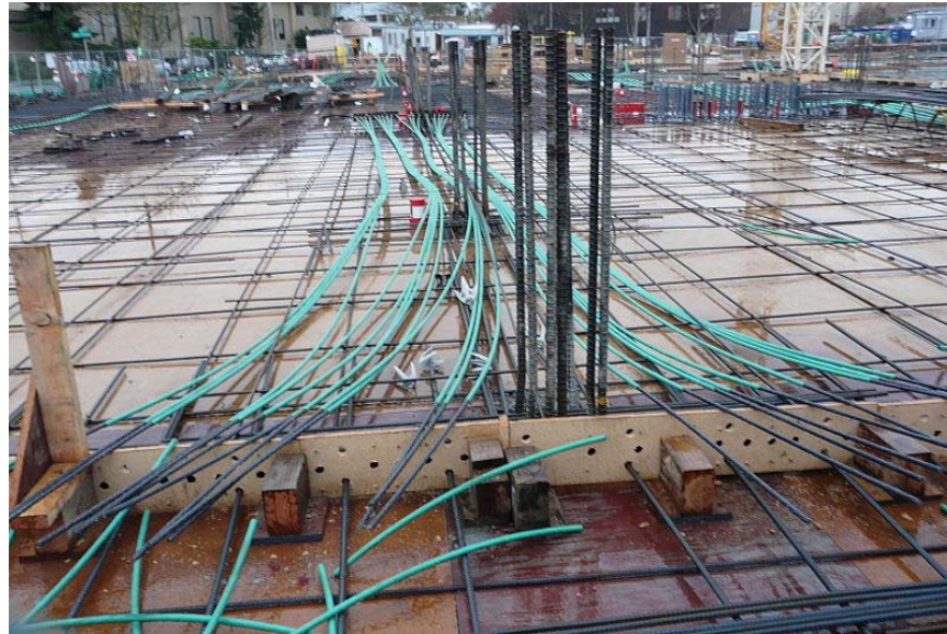
Figure 18: Two-way post-tensioned floor system ( www.wikipedia.com )
