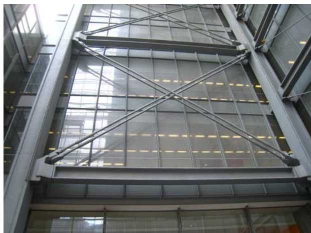
Figure 11: Exposed exterior X-braced rods
