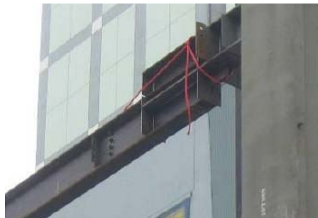
Figure 3: 'Dog-leg' beam connection, courtesy of Thornton Tomasetti
