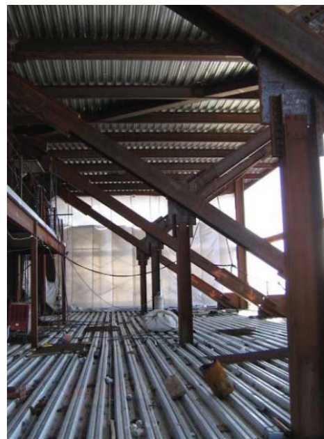
Figure 10: Outrigger bracing on mechanical floor
