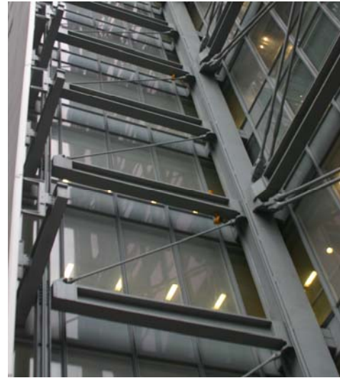
Figure 7: Cantilevered bays from exterior
