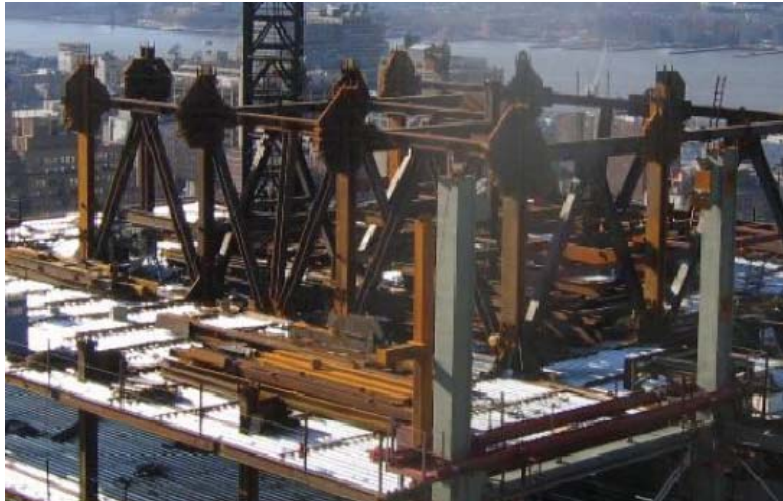
Figure 9: Core bracing during construction
