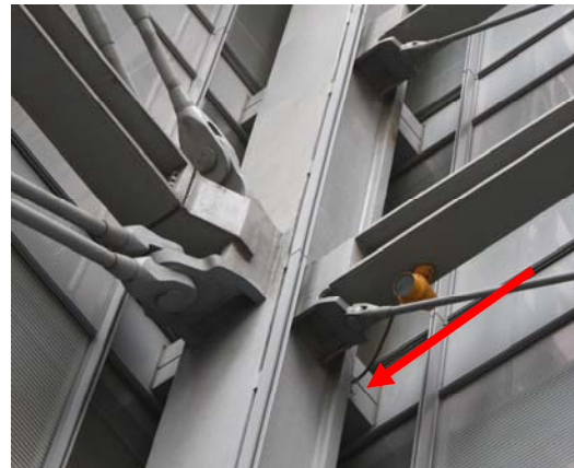
Figure 4: 'Dog-leg' penetrating building envelope
